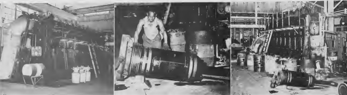
TWO GERMAN diesel generators helped power Lago's World War II effort. Diesels were DOS GENERADOR shown Alesan a yula duna forma pa e colozho di Lago den Segundo declared surplus with the addition of a steam generator at Powerhouse No. 2, Dismantling GERMA Muddal. E dieseln a ser deklará surplus tempo cu un generador di steam a ser instalá den Powerhouse No. 2. Nan a cuminsa desmantelanan na Juli de e huce mitsi began last July.
